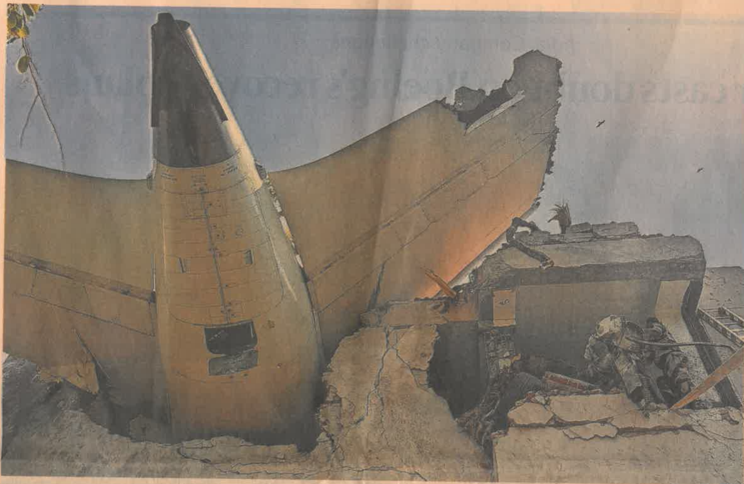
The rear of the plane protrudes from buildings in Ahmedabad: a survivor, said to be a Briton, walked away AFP Photo/Central Industrial Security Force
