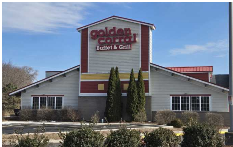
The owner of the former Golden Corral on Randall Road in Elgin wants to turn it into an Indian fusion restaurant and banquet hall. GLORIA CASAS/ THE COURIER-NEWS
