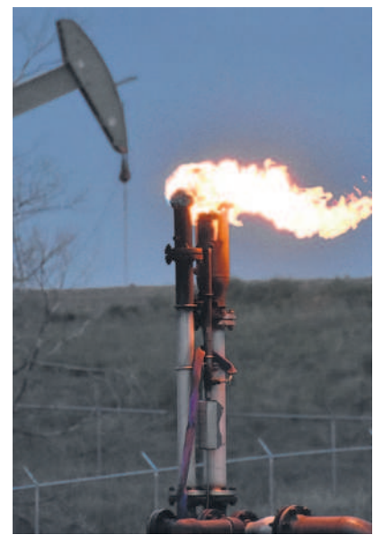
Gas flares sometimes let methane escape into the air
