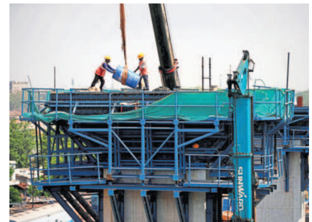
File photo of labourers at a construction site of the Ahmedabad-Mumbai High Speed Rail corridor in Ahmedabad. REUTERS
